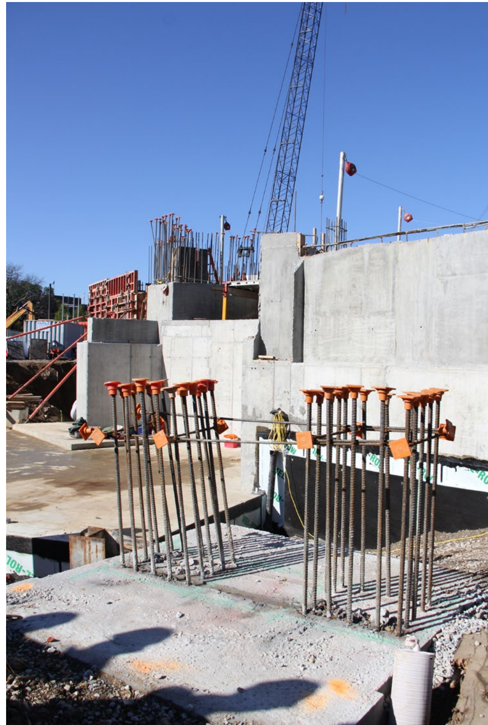
A "pad" foundation for a reinforced concrete column with continuity steel projecting
