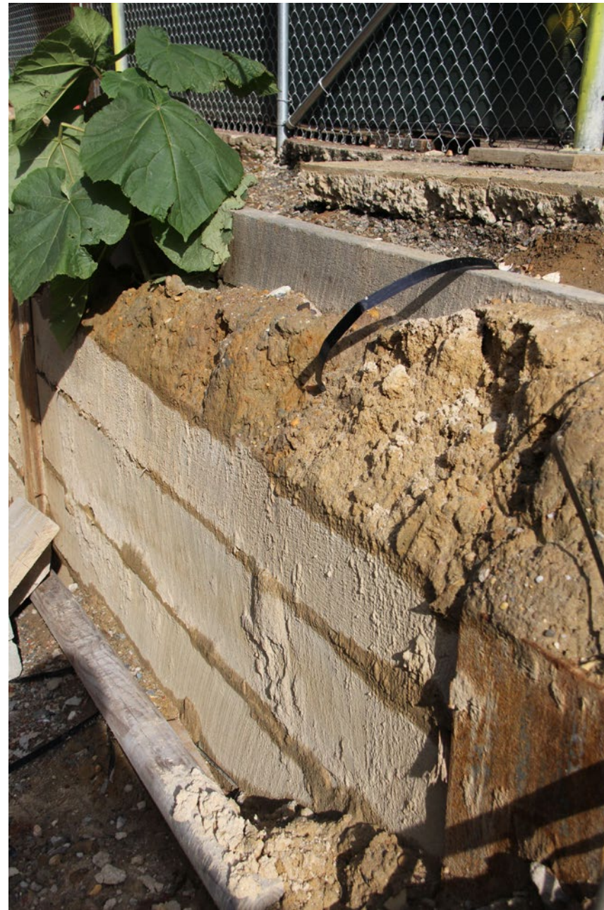
Temporary support system - Weak concrete retaining wall
