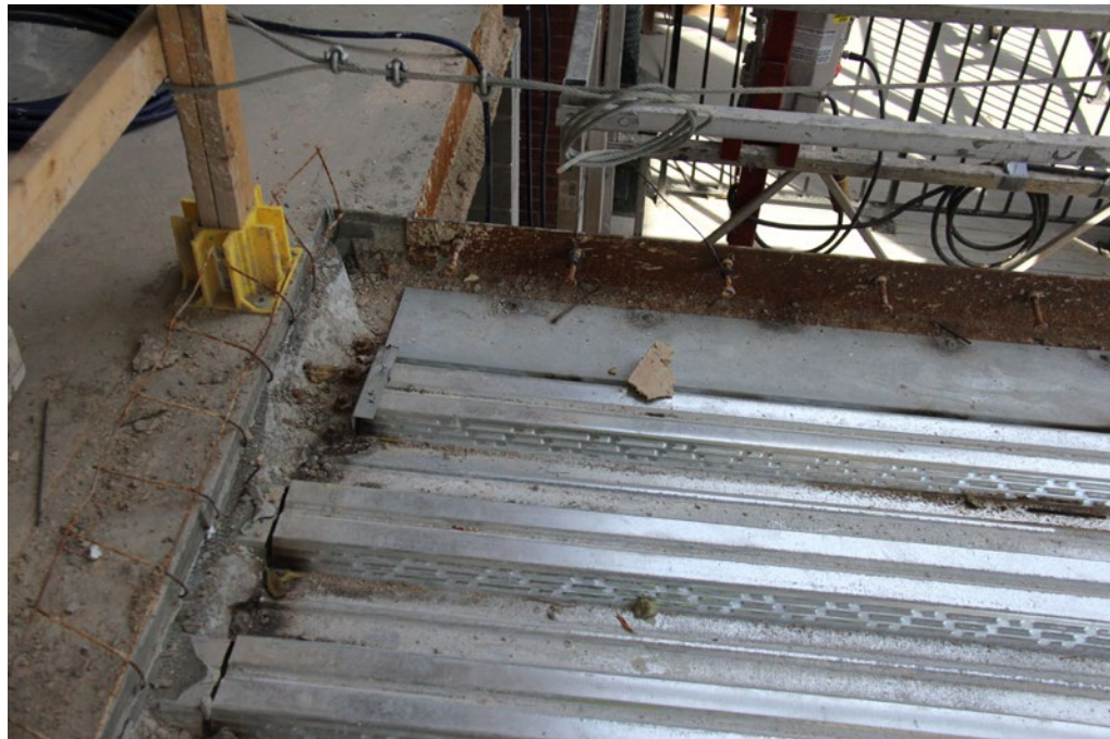
Steel edge angles welded on to top of edge beams to contain the concrete floor slab, from top of decking
