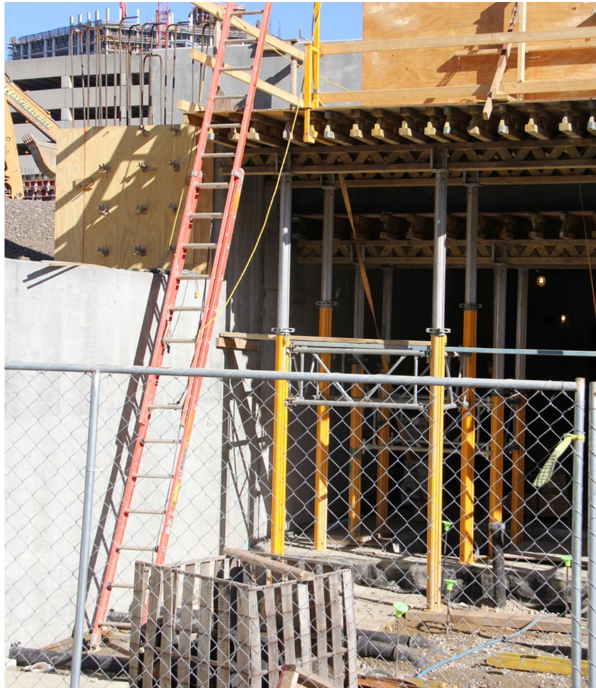
A reinforced concrete retaining wall after removal of the formwork (on the left hand side)
