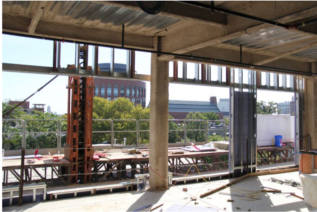
Fireproofing of columns with spray-on compound
