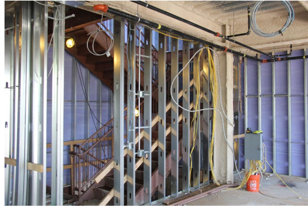
Fireproofing of columns with spray-on compound at the stairs
