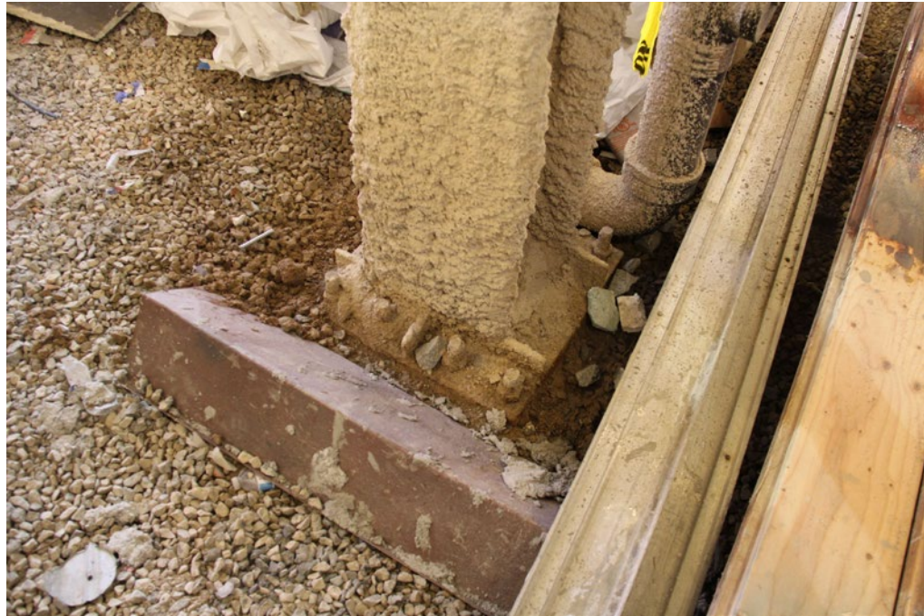
Column and baseplate to concrete foundation junction, with fireproof spray-on compound on column
