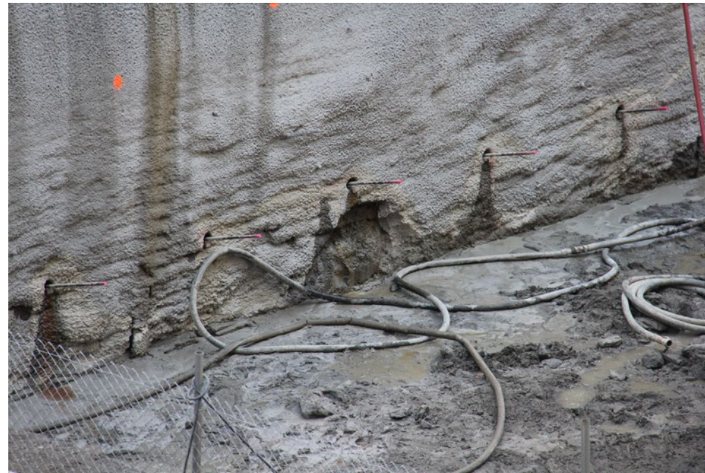
Temporary support system - Soil Nailing
