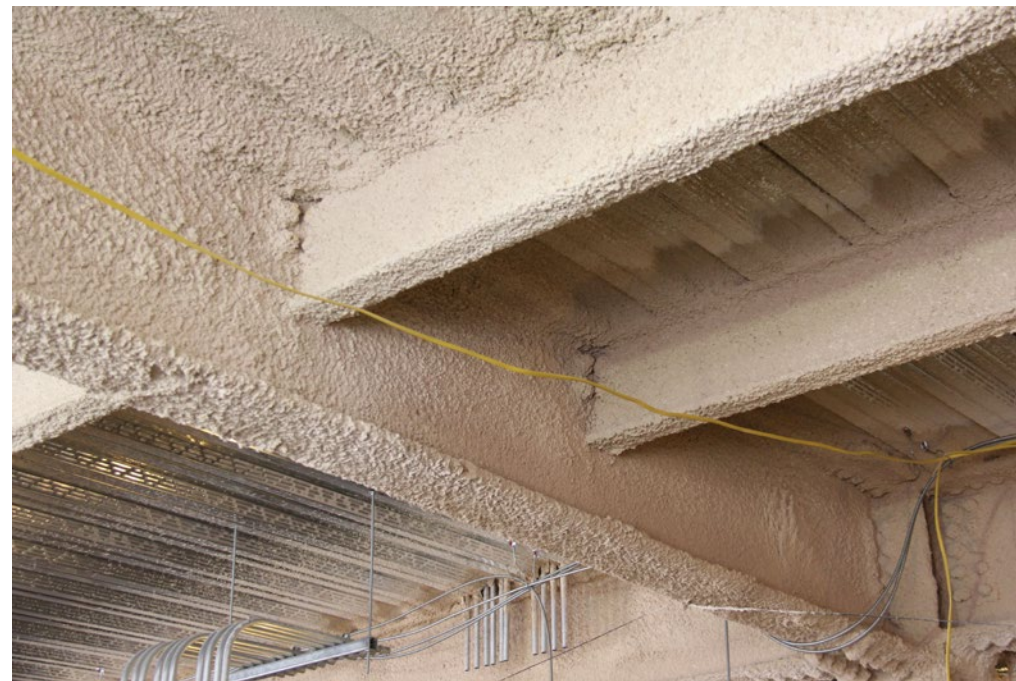
Secondary "floor support beams" to main girder junction, with fireproof spray-on compound
