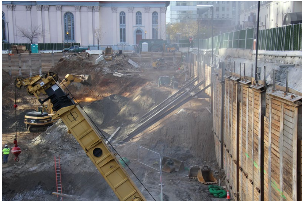
Temporary support system - Raker Bracing
