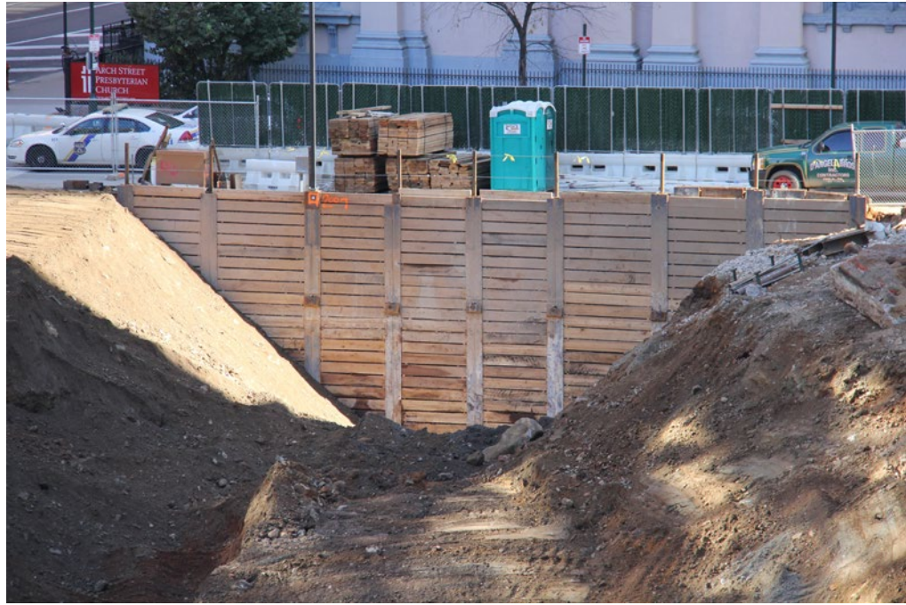
Temporary support system - Shoring
