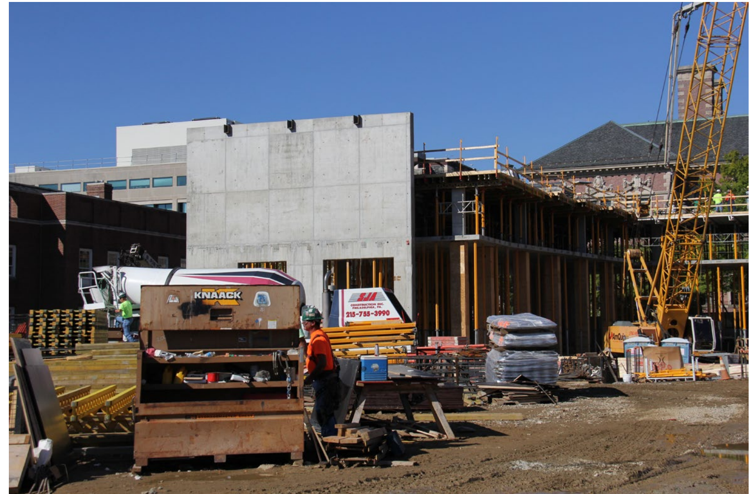
A reinforced concrete shear wall after removal of formwork
