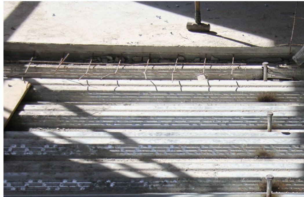
Concrete floor slab cast on to steel decking
