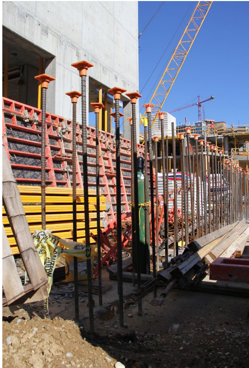
Strip Foundation with continuity steel reinforcement bars projecting
