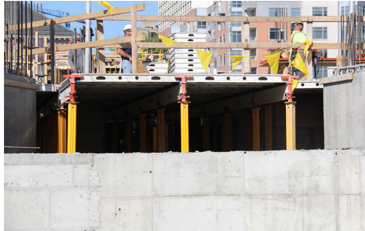
A “flat slab” construction
