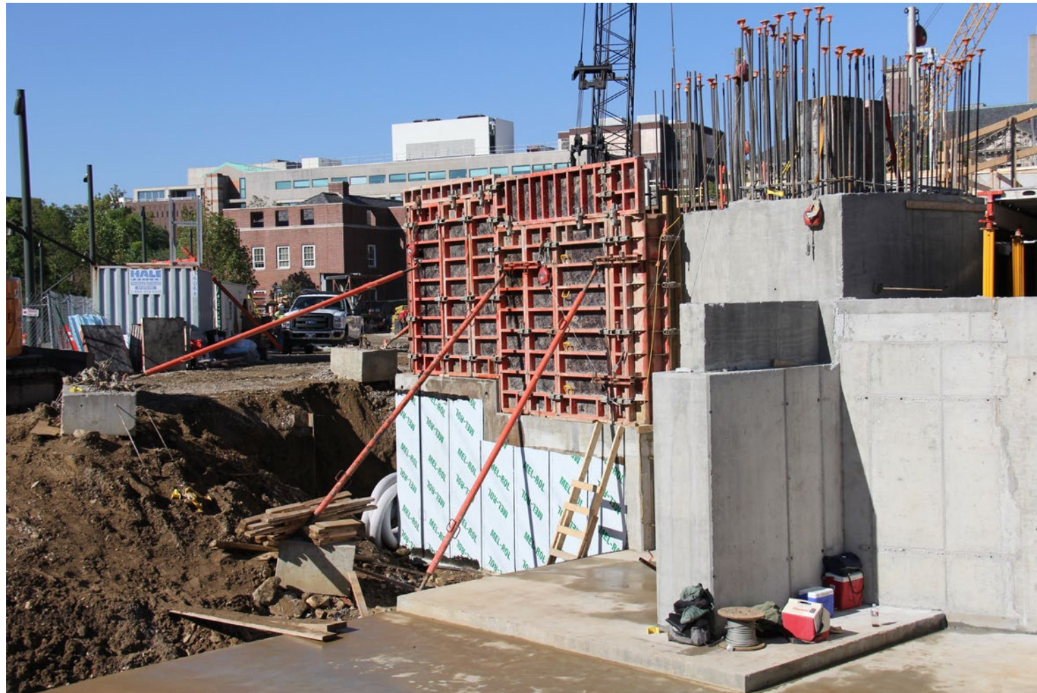
Formwork for a reinforced retaining wall
