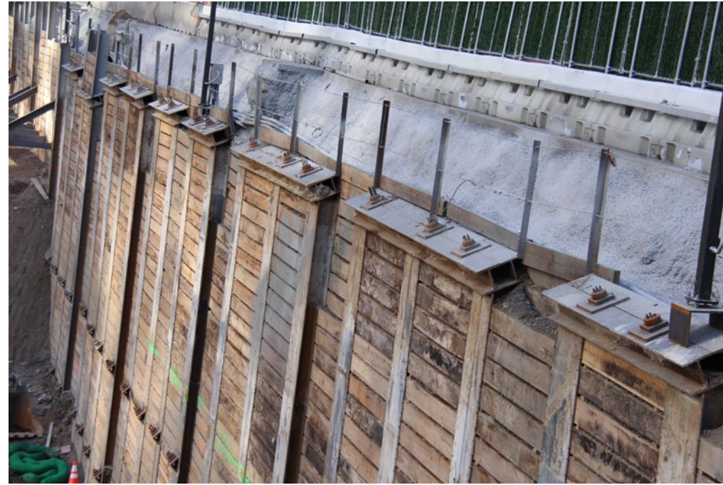
Temporary support system - H Piles
