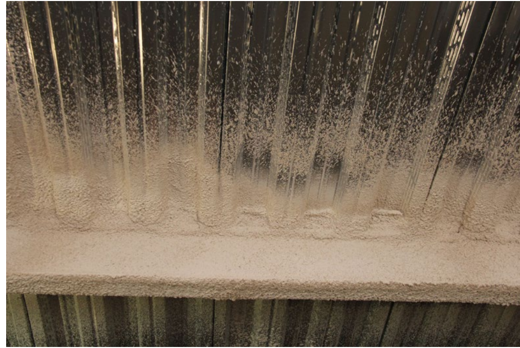
Closer view to the steel floor decking and support beam junction with fireproofing applied
