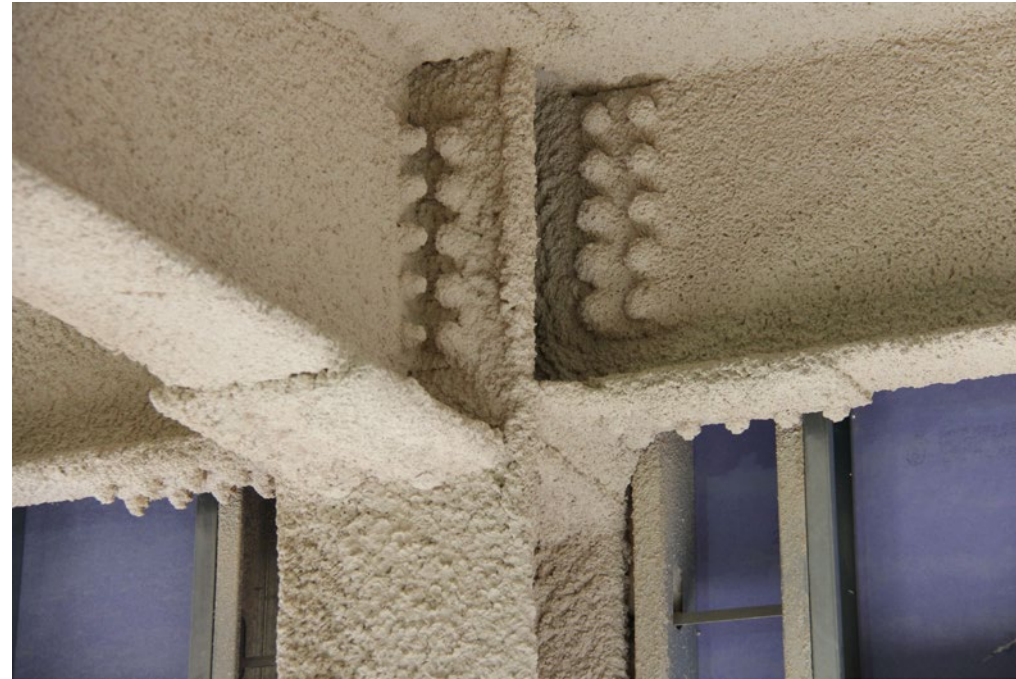
Main girder to column junction with fireproof spray-on compound
