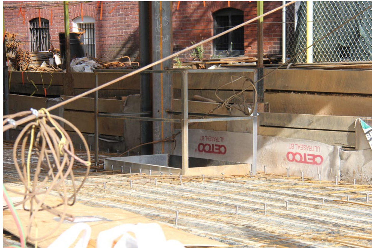
Temporary support system - Shoring (in the back)
