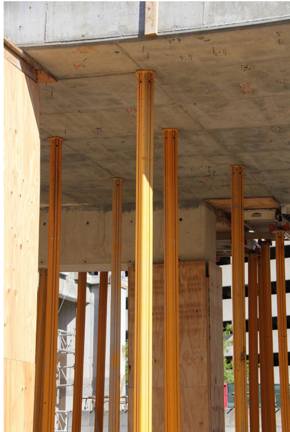
A "column to beam" connection with formwork attached
