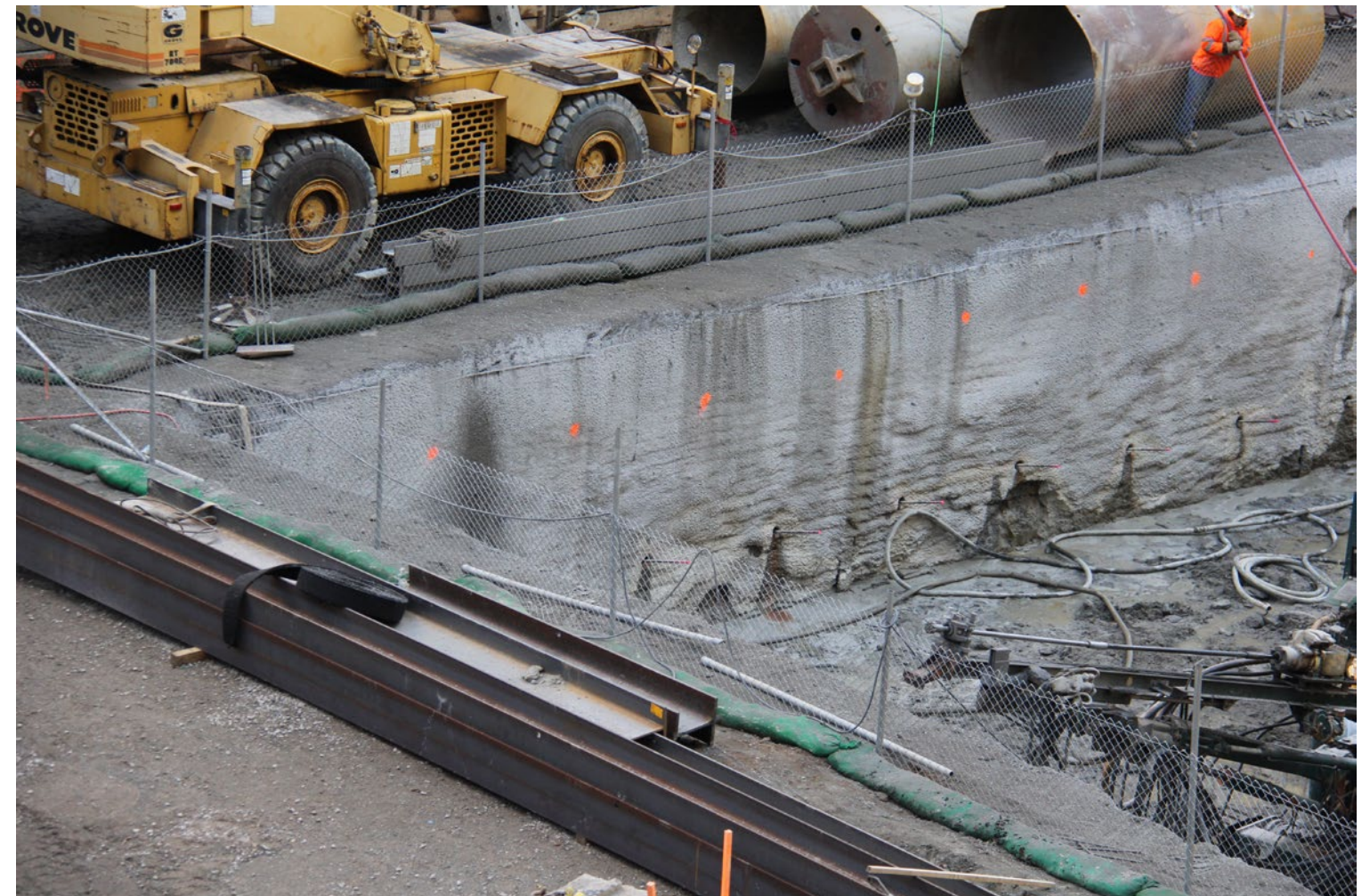
Reinforced concrete retaining wall to a deep basement
