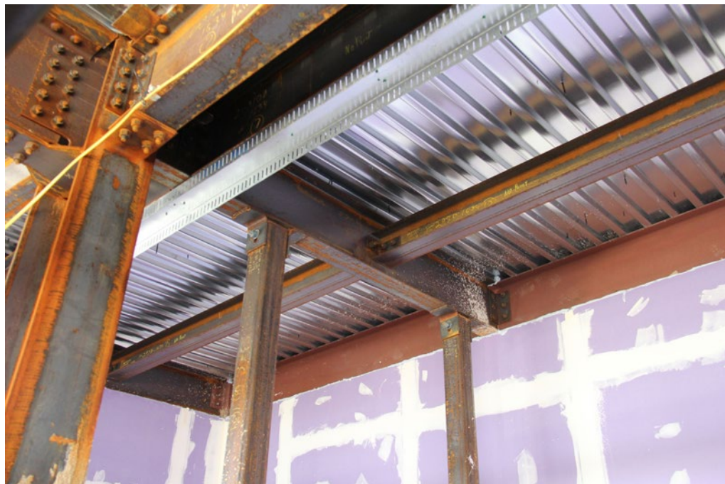
Steel floor decking with steel main girders and steel supporting beams
