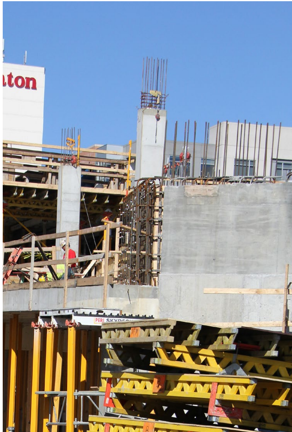
A reinforced concrete column after removal of the formwork
