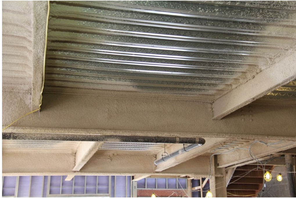
Steel floor decking to support beam junctions, from bottom of the deck
