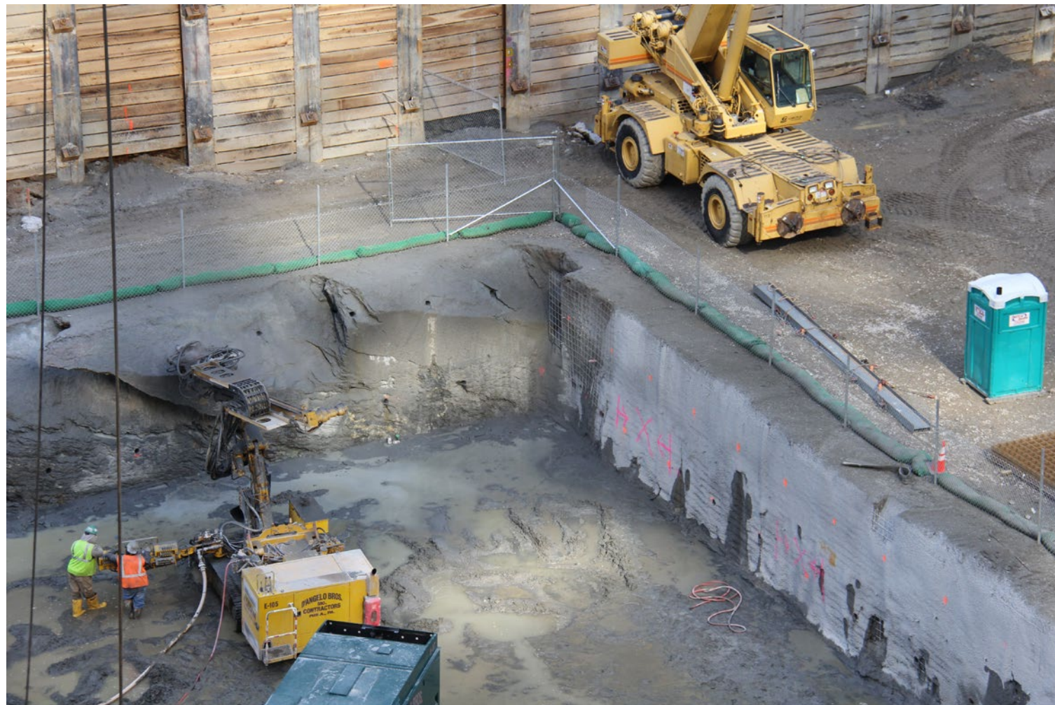
Reinforced concrete retaining wall to a deep basement
